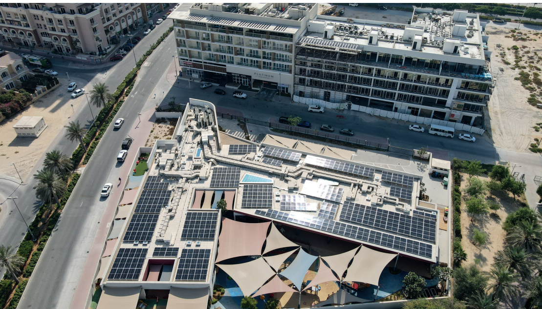
Arcadia High School JVT, Dubai 415.84 kWp
