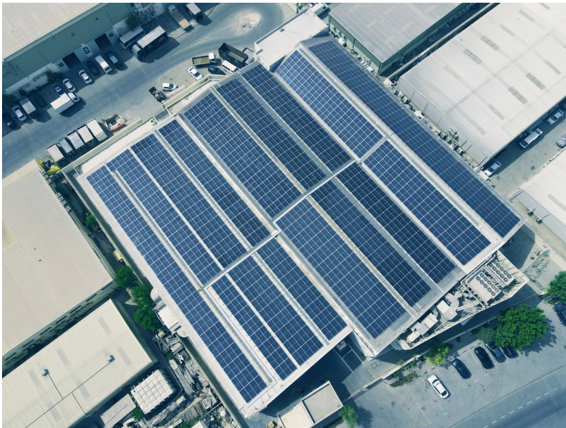
Emirates Printing Press Al Qouz Branch 610.4 kWp
