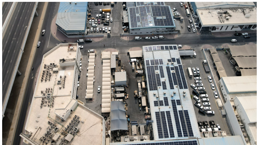
Scania Showroom Sheikh Zayed Road 530.28 kWp
